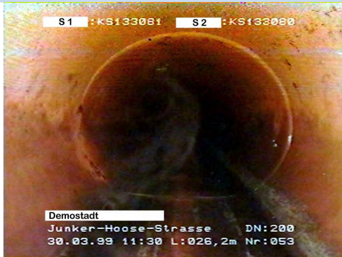
Deformation, Verformung
